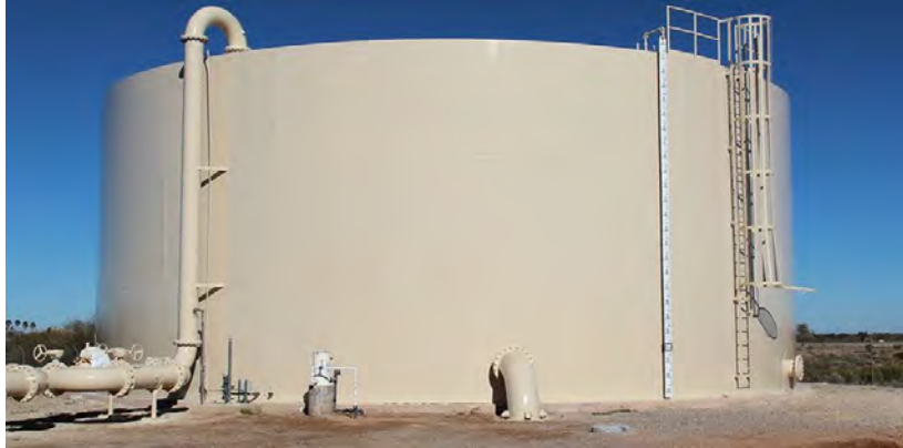
Figure 6 - Welded Steel Tank
