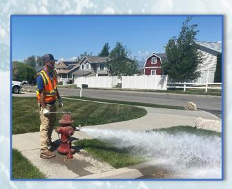
inside of the pipe wall stirring up sediments and breaking up deposits that can then be flushed out the opening of the hydrant. Flushing times for each hydrant will vary anywhere from 2-3 minutes up to 15-20 minutes depending on how quickly the flushed water clears up. Operators will complete testing of the hydrant by measuring available fire flow and water pressure at the hydrant.
