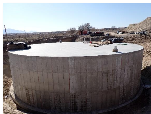
Image 3.) Construction of Buried Magna Water District Zone 3 Storage Tank.
